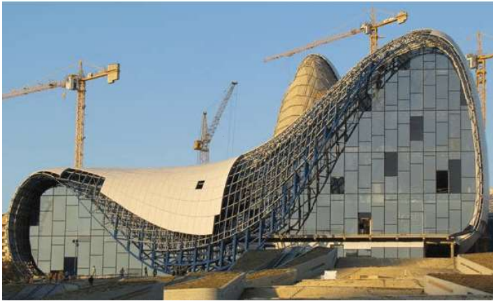
Figure 15 Assembly of the facade elements of the Heydar Cultural Centre in Baku. Each panel being unique for the particular part of the facade it belongs to. (Schielke, 2017)
