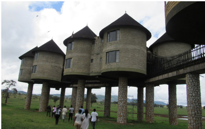
Fig. 5.113 The lodge accommodation units sit on stilts that resemble structural support in trees.
