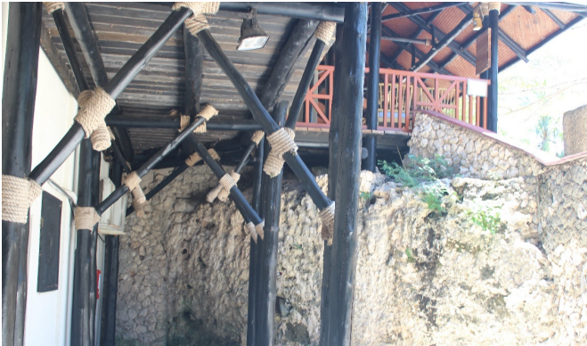
Fig. 5.153 The Coral Rock Café extends outdoors in to a cantilevered wooden deck that is supported off the cliff on tree like timber structure.
