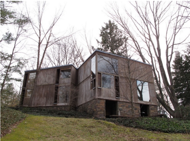
Fig. 3.64 Norman & Doris Fisher House (1967) by Louis Khan is a house finished in cedar wood cladding and masonry stone which bring a high aesthetic value due to the materials revealing the age and change the materials have undergone. Source: http://architectuul.com/architecture/fisher-house
