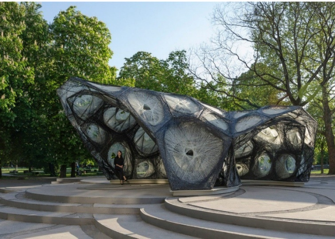
Fig. 3.62 ICD-ITKE Research Pavilion 2013-14 by ICD-ITKE University of Stuttgart is a biomimetic investigation of natural fiber composite shells and the development of novel robotic fabrication methods for fiber reinforced polymer structures. Source: https://www.archdaily.com/522408/icd-itke-research-pavilion-2015-icd-itke-university-of-stuttgart
