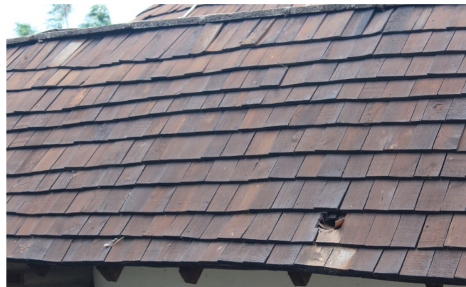
Fig. 5.114 The original timber shingles used on the roof reveal age and the change that the lodge has undergone.
