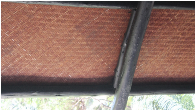
Fig. 5.163 Picture of woven coconut palm leaf soffit.
