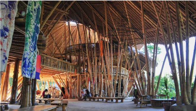
Fig. 3.59 A Bamboo Cathedral at Green School Bali in Bali, Indonesia structure mimics the natural tree structural support.
