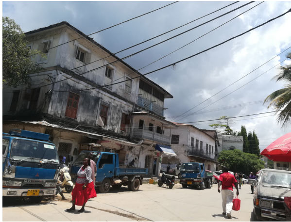
Fig: 1.12 Image showing the external lime plaster affected by weather elements on mkunazini street. Source: Author, (2018).
