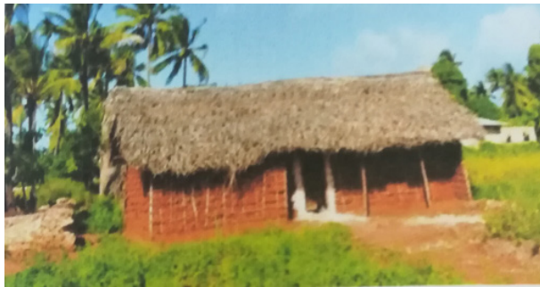
Fig 1.26 Image showing makuti used on the roof Source: Author (2018)
