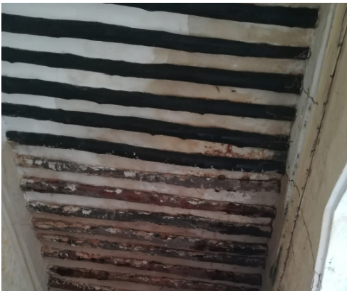
Fig 1.24 Image showing mangrove poles used on the ceiling. Source: Author (2018)
