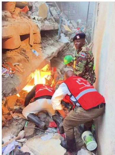
Figure 1-2 Collapsed in the early hours of Tuesday, 12 May 2015 in Nairobi Huruma Estate after floods and torrential rain.
